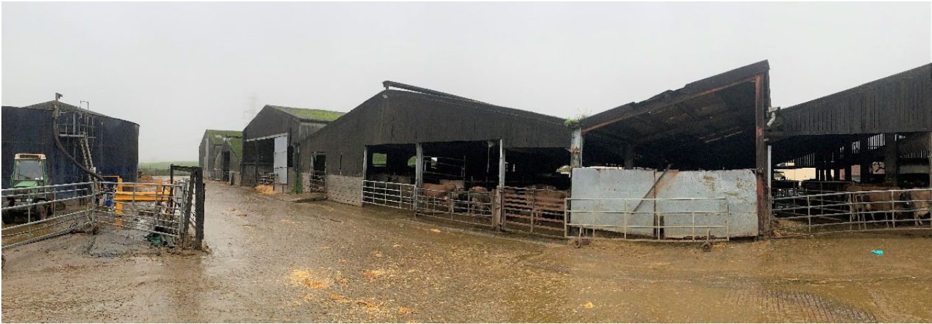
Photos 1 - 4: Some of the Dairy Buildings
